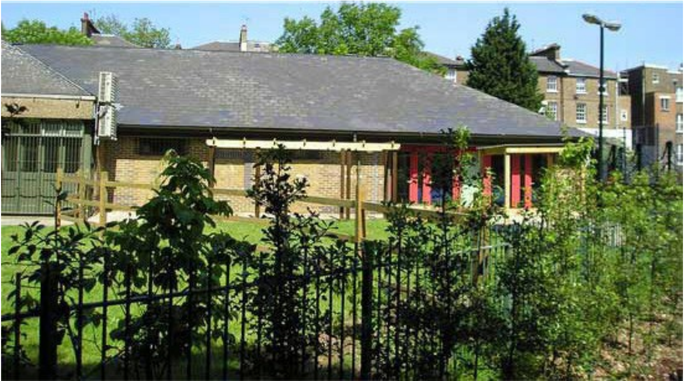
Hilldrop Community Centre (Source: Hilldrop Community Centre)
